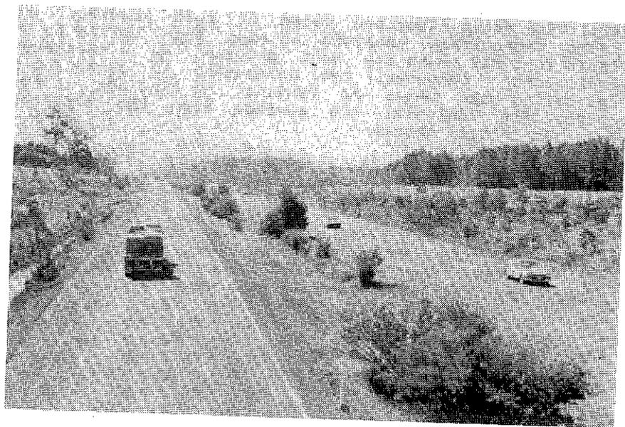
Photograph 2: The standard of facility with opposing traffic separated by 10m wide reserves which could have been built fifteen years earlier if the strategy suggested in this paper has been implemented.
