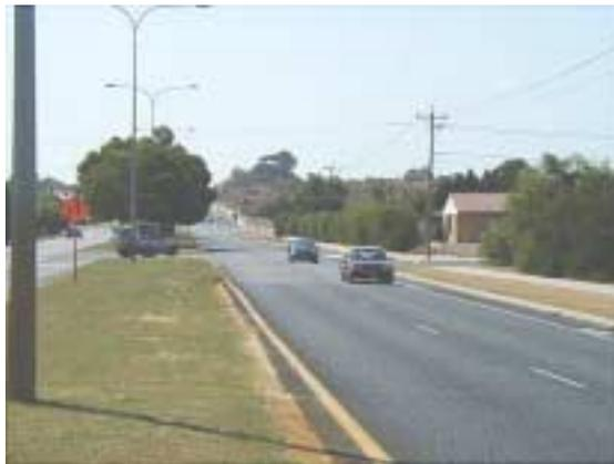
Figure Five: Four lane Divided Distributor without driveway access
