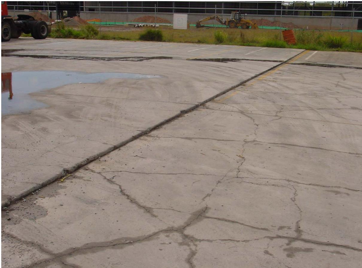
**Figure 2**      **Detail of 65mm drop in level between warehouse slab and manoeuvring apron.**
