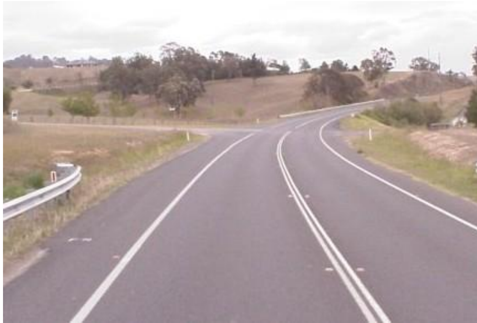
Image 3 - Typical 800 metre radius curve on a two lane rural road
