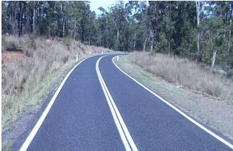
Image1 - Typical 300 metres radius curve on a two lane rural road
