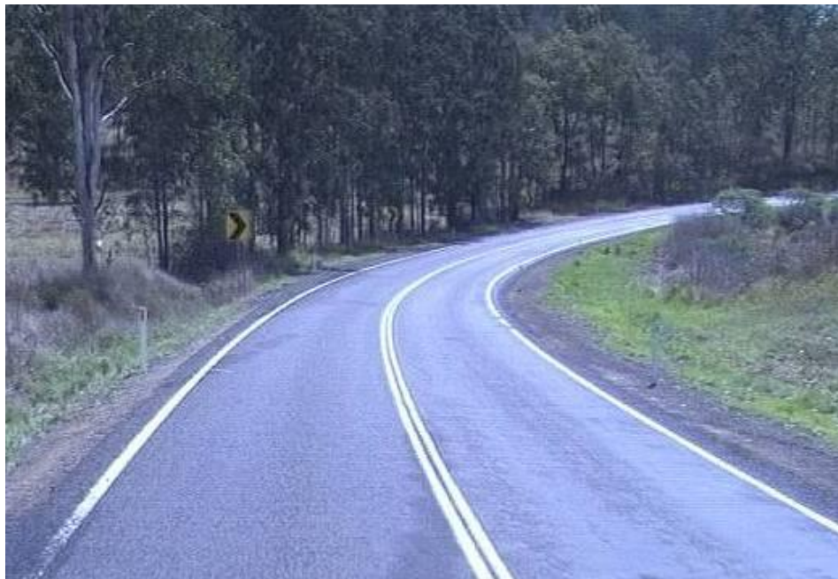
Image 2 - Typical 150 metres radius curve on a two lane rural road – Note the Curve Alignment Markers
