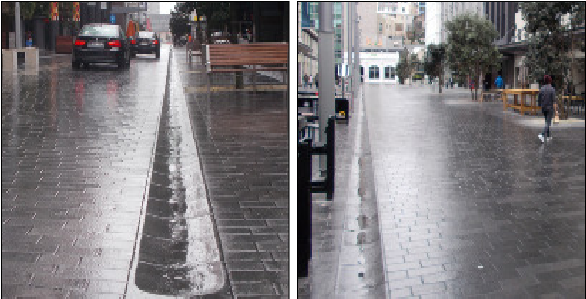
Figure 7: Drainage Channel Alongside Circulation Zone – Federal St and Fort St (east)
